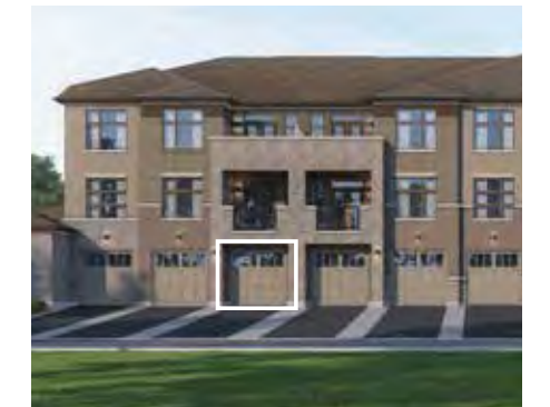
REAR, Interior Unit
